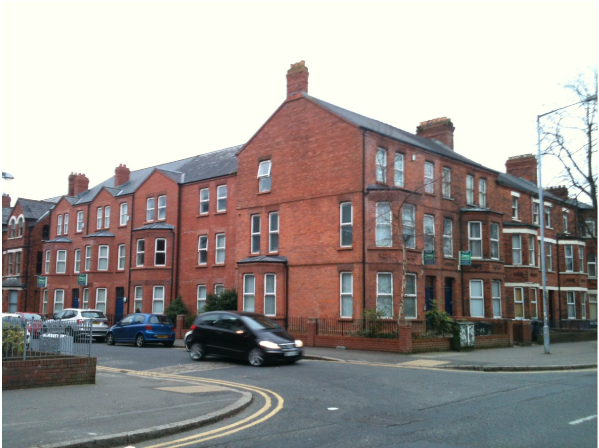
Corner Eglantine Gardens / Eglantine Place
